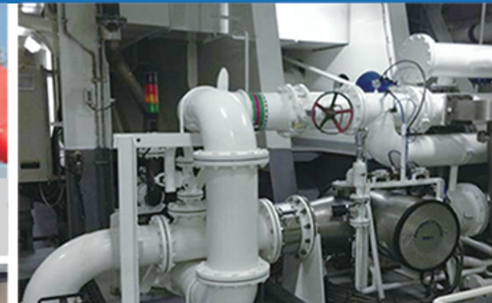
Ship Owner □ Germany (CP Offen) | Ship Type □ 4100TEU Container Pump Capacity □ 500m 3 / h x 2 | Model □ BSKY500 x 1 set Skid Type Class □ GL
